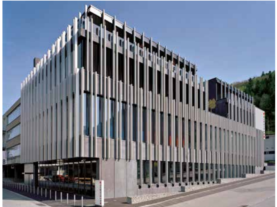
Built corporate identity: the facade of the corporate headquarters in Littau near Lucerne features vertical aluminium pilaster strips that form an excellent point of reference with our products and market partners.
